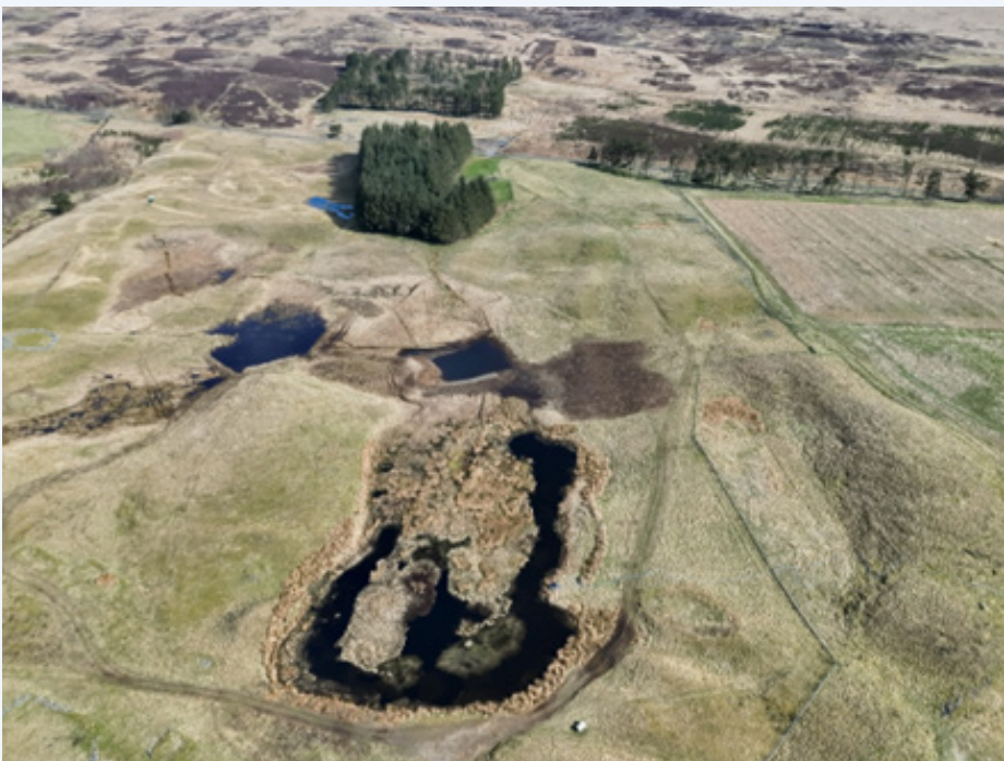
Figure 14: The existing pool at Wheen is shown in the foreground in figure 14. Newly created pool and wetted areas behind new bunds can be seen in the background.
