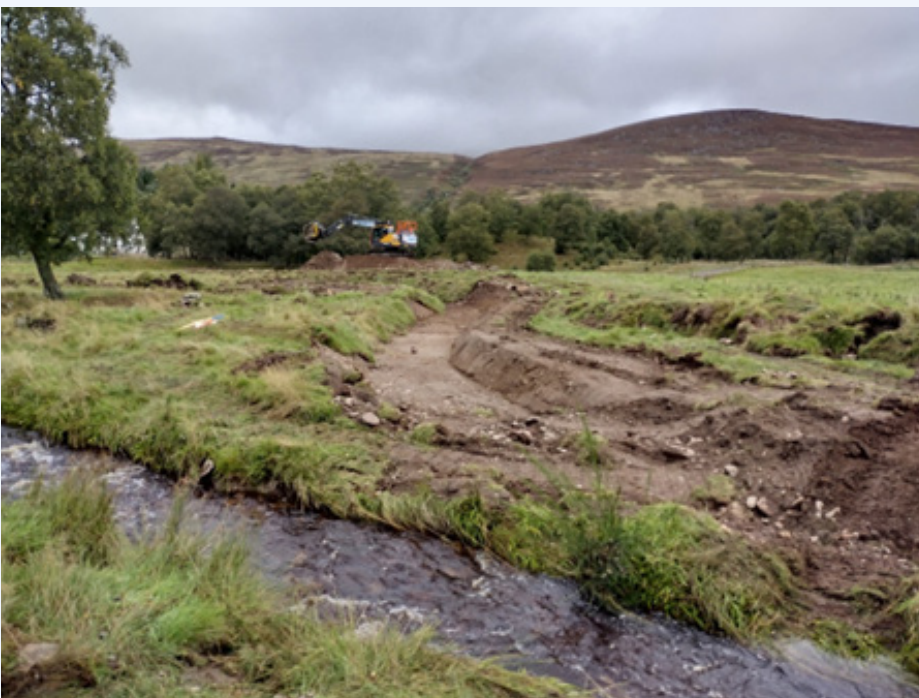
Figure 2: Creating the new channel began in September 2025. Figure two shows a digger onsite excavating the new March Burn channel with the original, straightened channel in the foreground.
