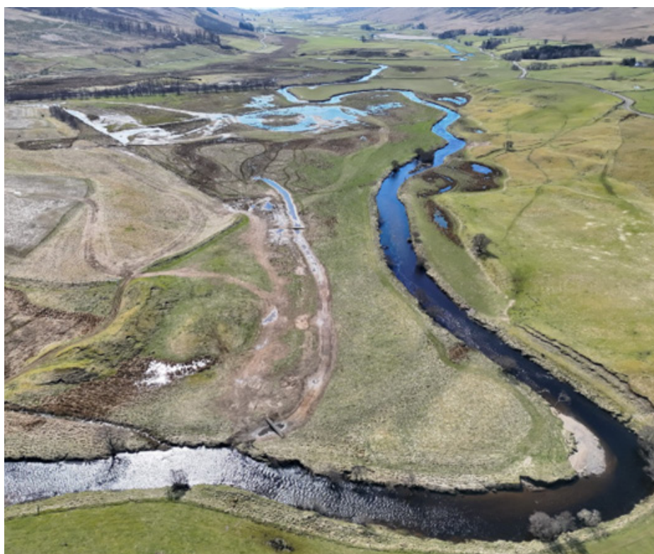
Figure 7 Laird's Haugh wetland site in April 2026, post-construction is shown in figure seven. Water is being held back on the floodplain in the southeastern end of the site.
