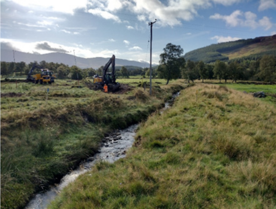
Figure 1: Construction phase began on site at March Burn in September 2025. Figure one shows a digger onsite prior to excavation of the original channel.
