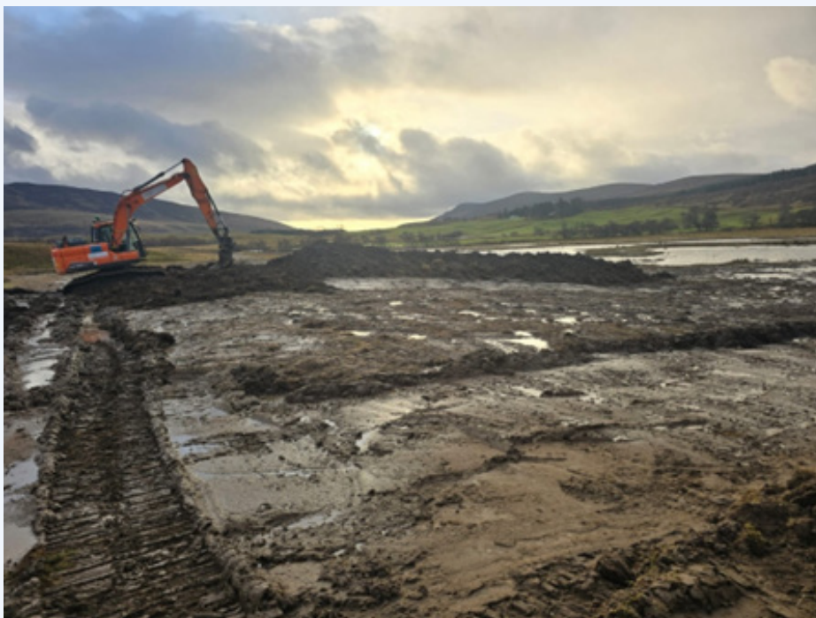
Figure 6: A digger on-site at Adielinn excavating the southern end of the offtake channel, where it meets the scrape cluster is shown in figure six.
