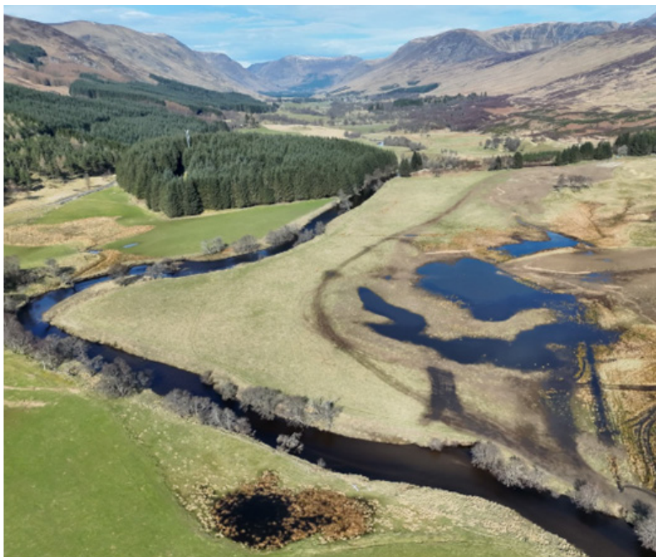
Figure 4: Adielinn wetland site in April 2026 post-construction is shown in figure four. Water is being retained in several of the newly formed wetland features and will vary in sync with rainfall in the upper catchment.
