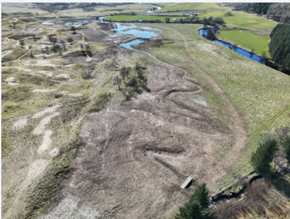
Figure 7: A drone image of the completed Adielinn wetland looking south-east is shown in figure seven. The vehicle access bridge, offtake channel are visible in the foreground. The cluster of scrapes and newly wetted areas behind bunds are visible in the background.
