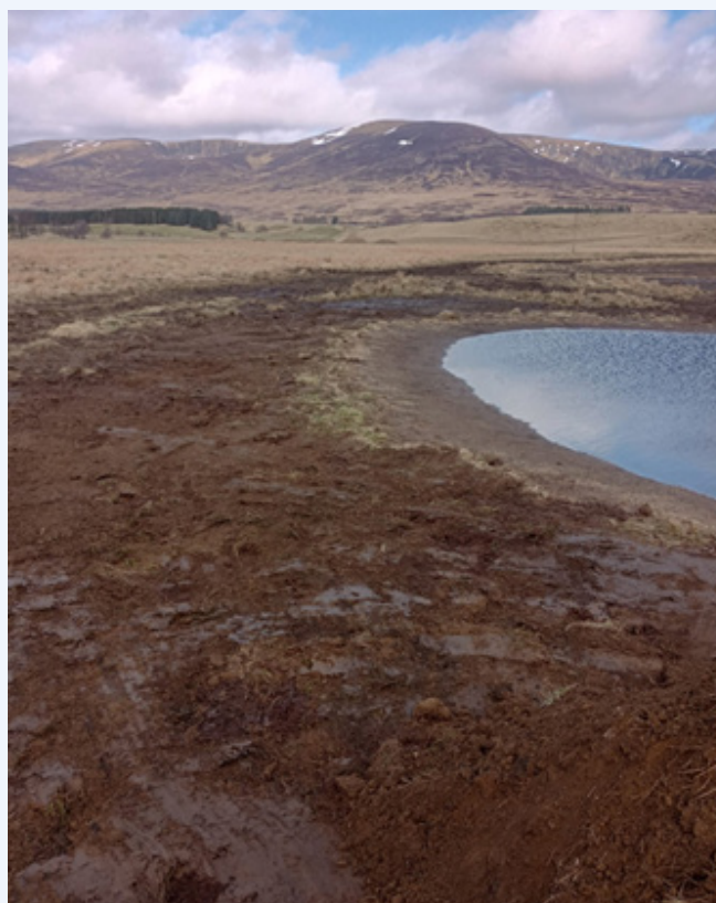
Figure 10: Looking east at Laird's Haugh, figure 10 shows a completed pool at Laird's Haugh. It highlights the purposefully constructed shallow edge, designed to support breeding wading birds.
