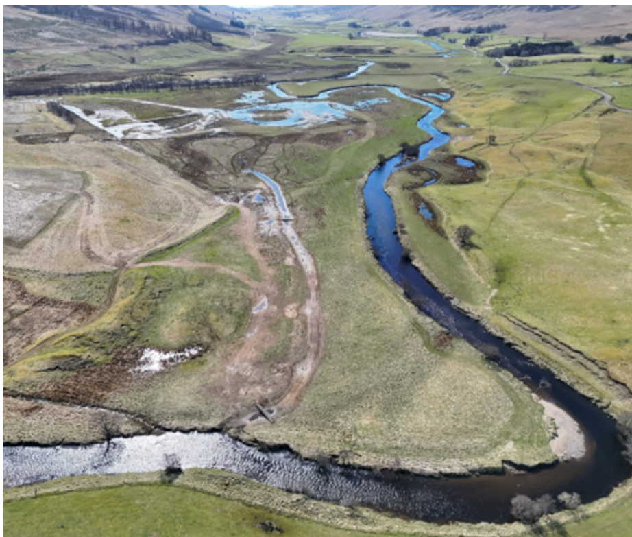
Figure 7 Laird's Haugh wetland site in April 2026, post-construction is shown in figure seven. Water is being held back on the floodplain in the southeastern end of the site.
