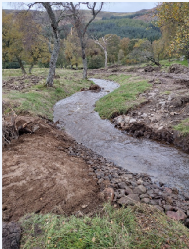
Figure 3: A section of the newly re-profiled riverbank and March Burn in the southern area of the site is shown in figure three.
