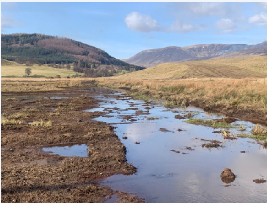
Figure 9: Looking north at Laird's Haugh, figure nine shows a re-profiled ditch which had been excavated by a digger.
